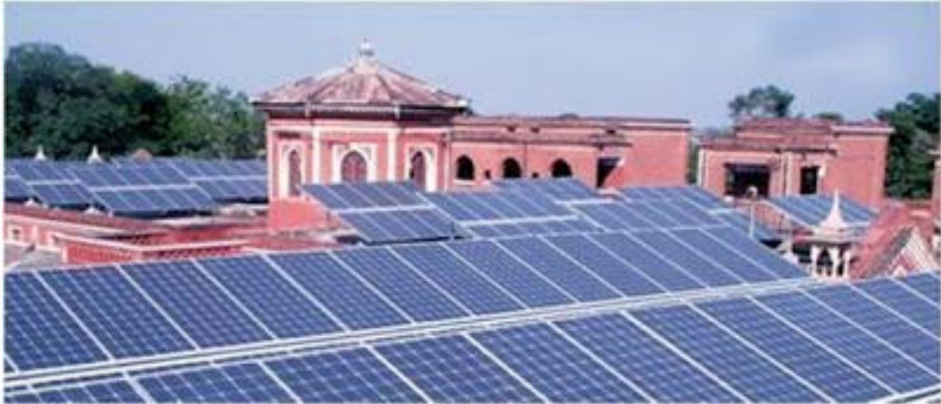
Roof top solar panels
